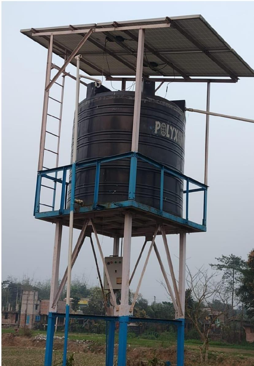
Figure 3: Solar power based backup water pump, Siddhinath Mahavidyalaya
