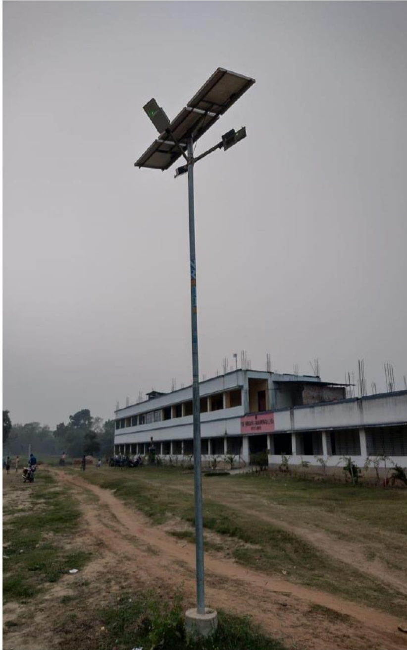
Figure 2: Solar panel based outdoor lighting, Siddhinath Mahavidyalaya
